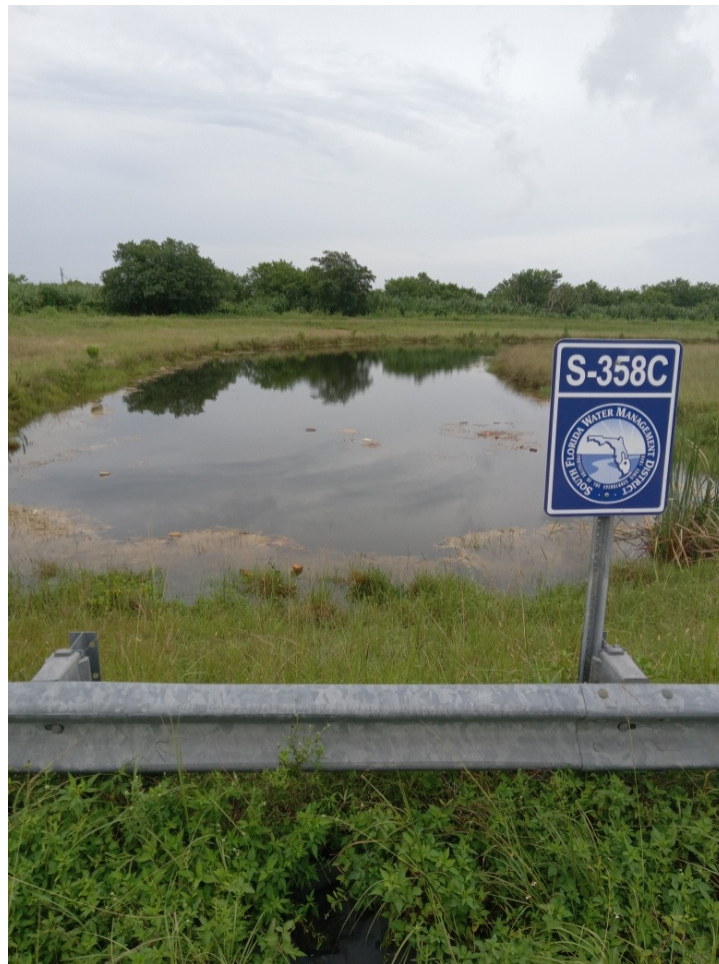
Cell phone photograph depicting South Florida Water Management District structure marker S-358C and surrounding water conditions.
