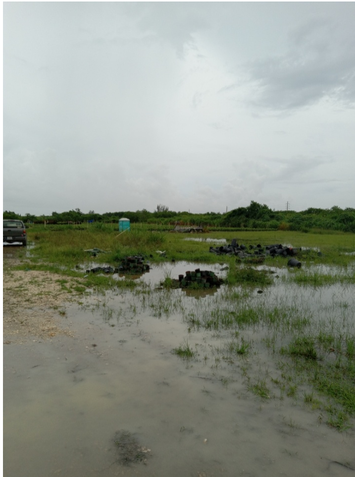
Cell phone photograph depicting standing water/flooding conditions affecting the field area.
