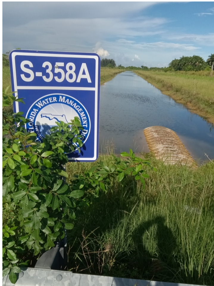
Cell phone photograph depicting South Florida Water Management District structure marker S-358A and adjacent canal/water conditions.
